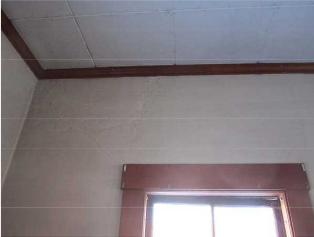
Stress cracks in plaster work have been previously repaired at northeast corner of meeting hall
