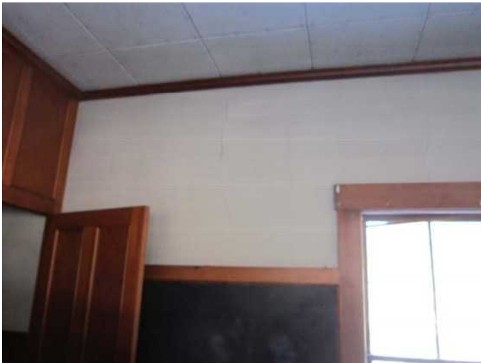
Minor cracking of plaster typical of foundation movement under frost action.
