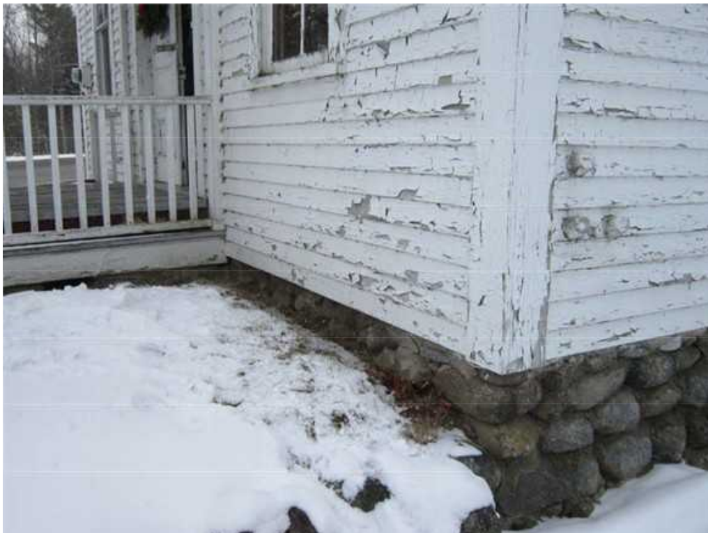
North east corner of main block showing extreme paint degradation and stone foundation
