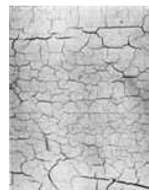
Crazing—or surface cracking—is an exterior surface condition which can be successfully treated by sanding and painting. Photo: Courtesy, National Decorating Products Association.
