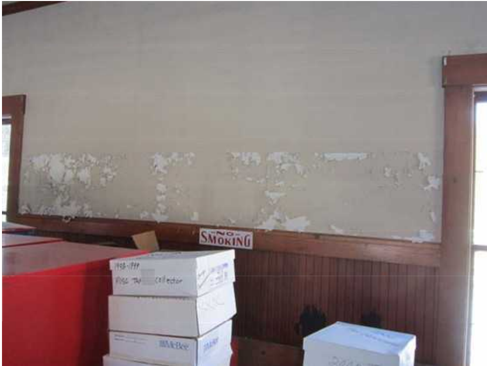
Localized area of paint failure behind where chalkboard or bulletin board was previously removed
