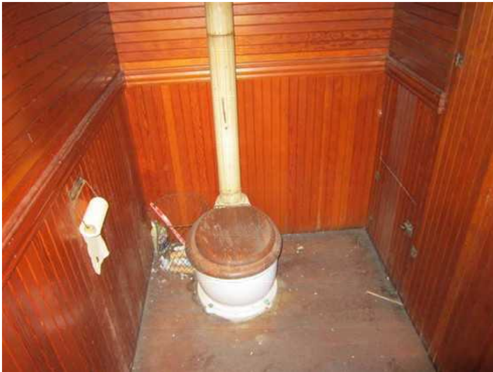
Privies are no longer working. Note that no plumbing in this bathroom impact the original wall finishes.
