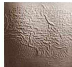
Wrinkled layers can generally be removed by scraping and sanding as opposed to total paint removal. Photo: Courtesy, National Decorating Products Association.
