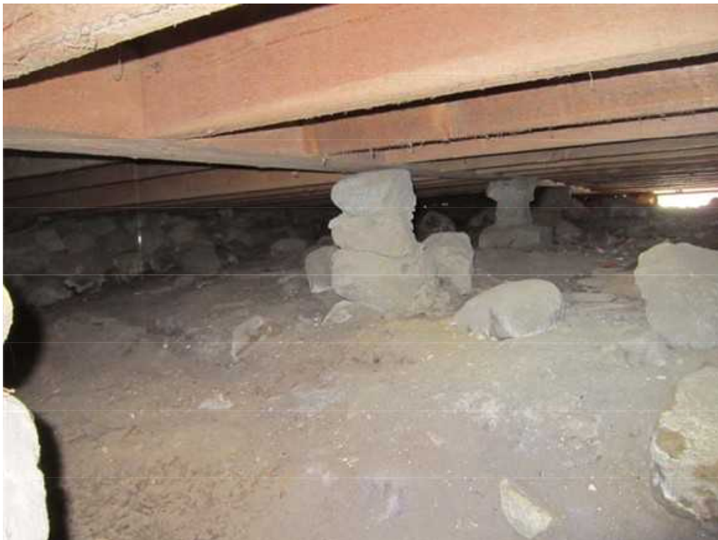
Existing crawl space with stone supports under beam - note proximity of floor framing to soil and complete lack of insulation in floor system above.
