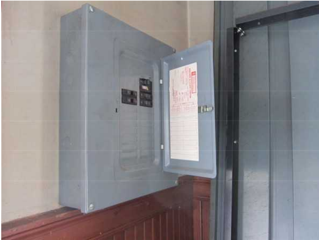
Circuit breaker panel. Most electrical work appears to have been updated in the 1980s, and other new wiring installed ad-hoc.
